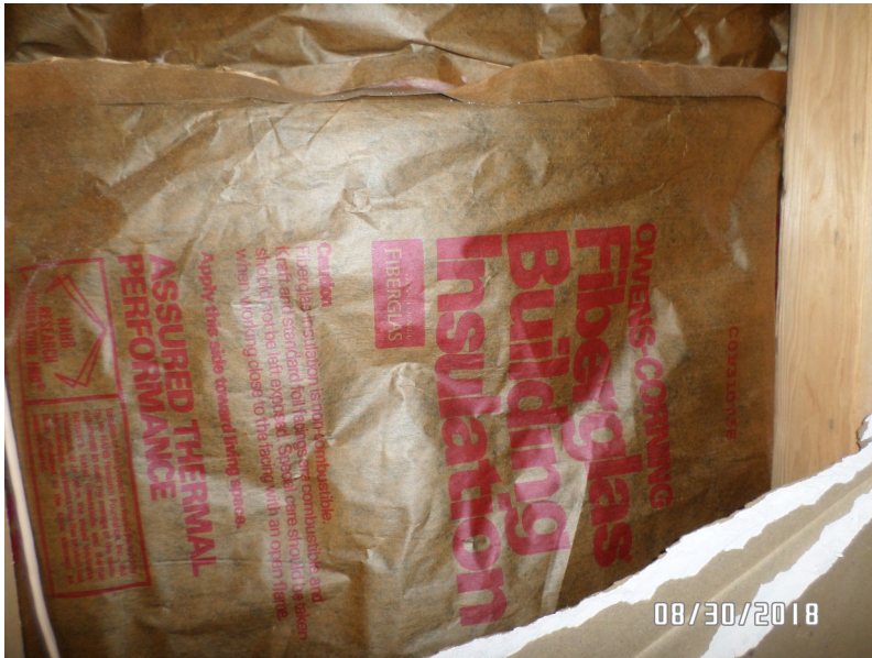
#7 - View of fiberglass insulation in walls of main level
