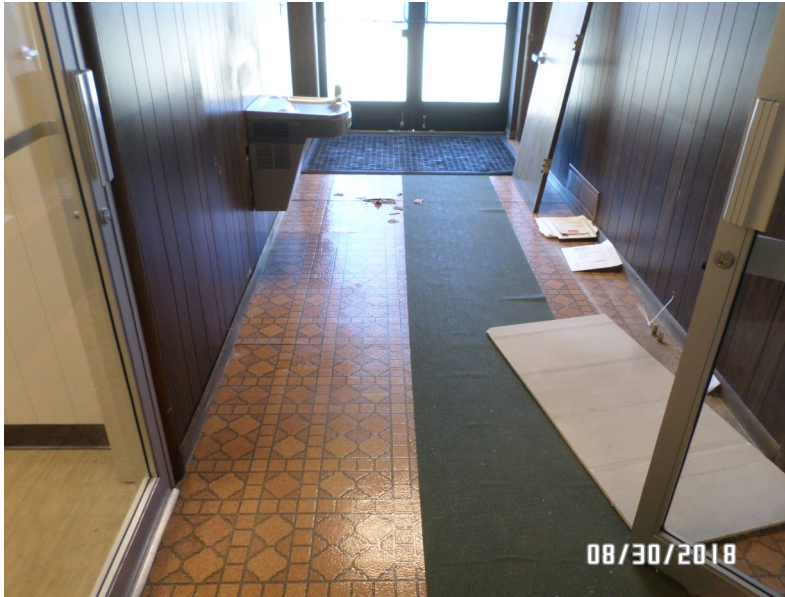
#9 - View of linoleum ACM (HM-4) at southwest entrance to structure
