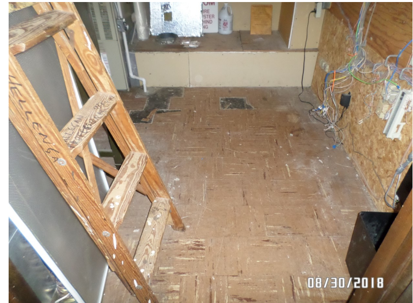
#12 - View of floor tile (HM-23 & HM-24) in basement of structure
