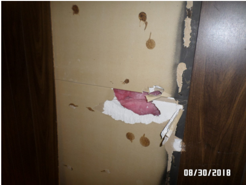
#15 - View of fiberglass insulation in walls of basement level
