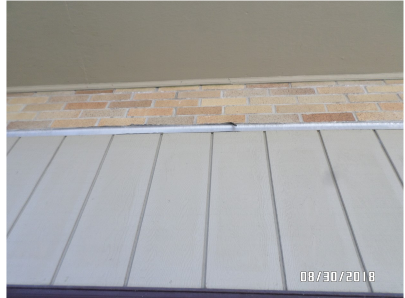
#26 - View of caulking (HM-29) between weather stripping and brick on north and west building facade
