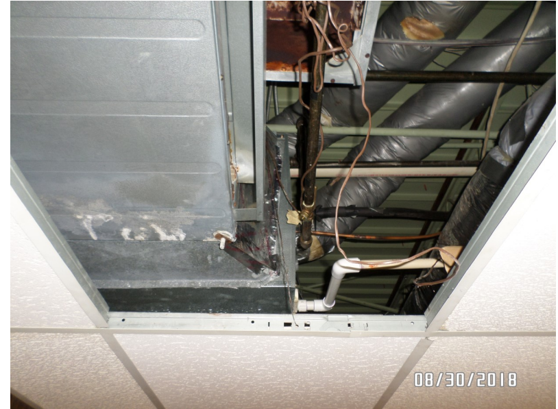
#10 - View of fiberglass insulated duct work and air supply piping above ceiling in main level
