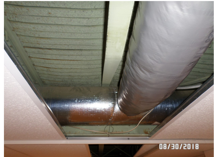
#16 - View of fiberglass insulated air supply piping in basement
