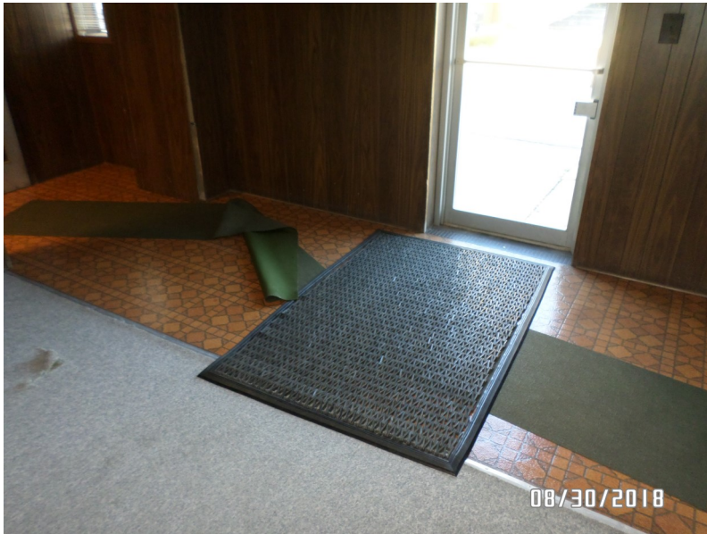
#3 - View of linoleum ACM (HM-4) at north entrance to structure
