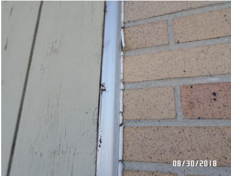
#25 - View of caulk (HM-27) between wood and brick on north and west building facade
