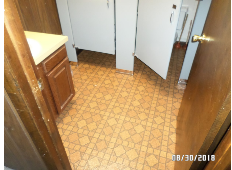
#18 - View of linoleum ACM (HM-21) in southern men's room in basement
