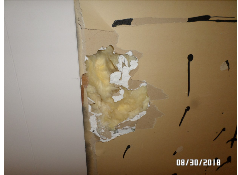
#6 - View of fiberglass insulation in walls of main level
